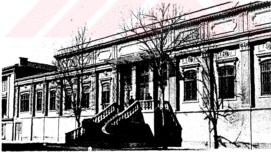
Figure: 4.21. Sanayi-i Nefise Building, 1883, by Vallaury.
