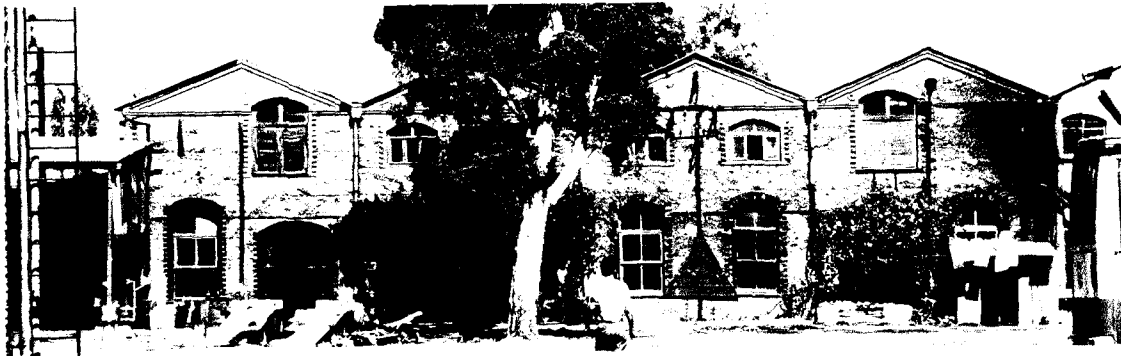
Figure: 5.21. The Gas Factory, Details
