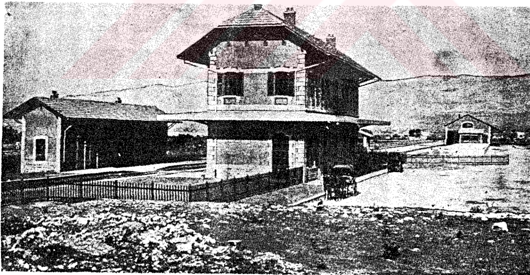
Figure: 4.48. Beirut Railroad Station, 1890, Constructed by a German Company.
