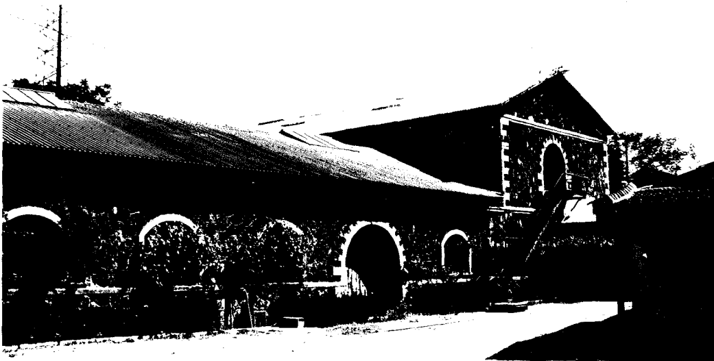
Figure: 5.27. The Punta Train Station, Repairing Buildings
