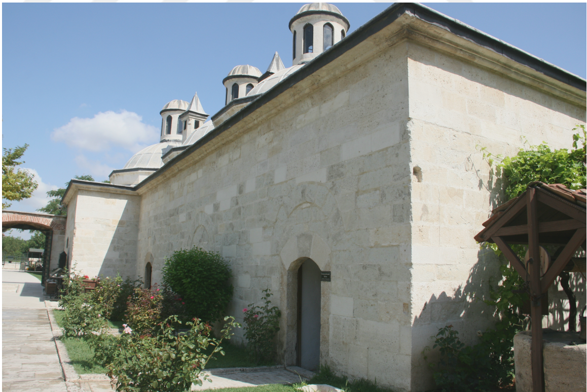
Figure 50: Rooms in the North east wing of the Bayezid II Darussifa. . Source: Author’s photograph.
