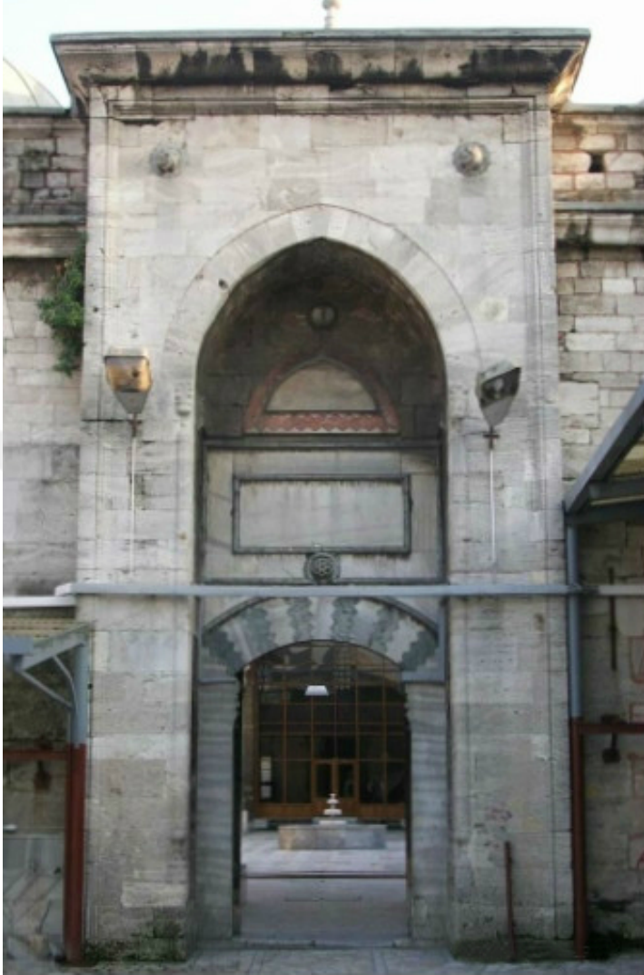
Figure 37: Main gate of the Fatih Tabhane, which is currently under construction. Source: www.formgrup.com
