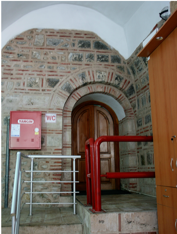
Figure 25: Eastern part of the classroom converted into a bathroom. Author's photograph.
