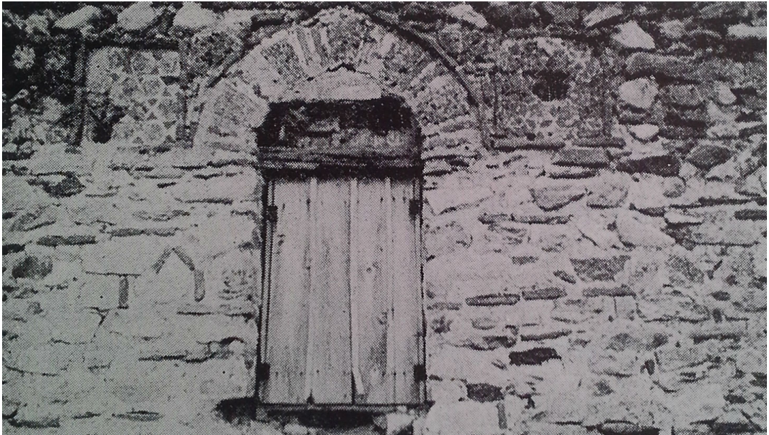
Figure 19: One of the west wing windows and the decorative panels, which no longer exist today. Source: Ekrem Hakki Ayverdi.
