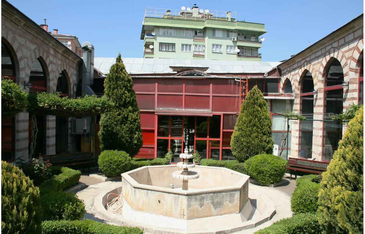
Figure 24: The Yıldırım Bayezid Darüşşifa Main entrance and northern iwans covered by metal construction and glass additions. Source: Author's photograph.
