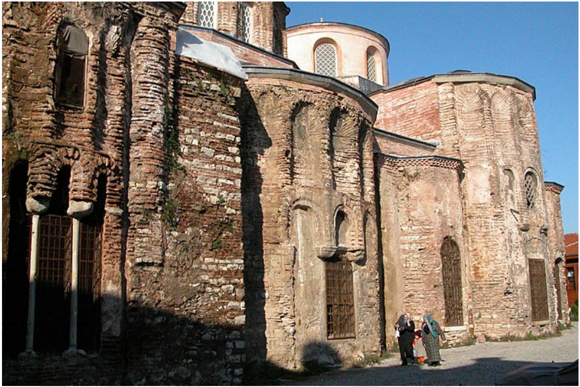
Figure 3: Exterior of the apses of the Pantokrator Church prior to the restoration. Source: ArtServe - The Australian National University ( http://www.pallasweb.com/ ).
