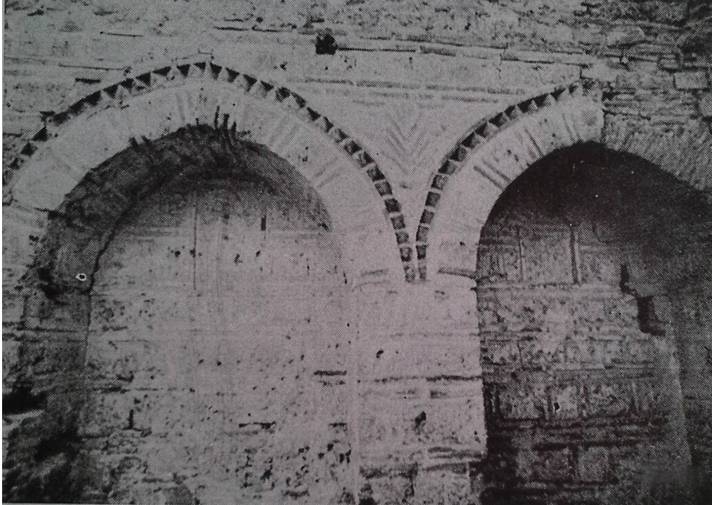
Figure 21: Decorative motifs on the western wall of the entrance gallery of the Yıldırım Bayezid Darüşşifa (1962). Source: Ekrem Hakki Ayverdi.
