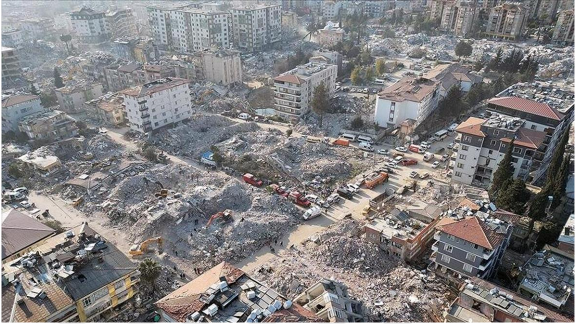
Figure 1: Kahramanmaraş earthquake (February 2023), Türkiye.
