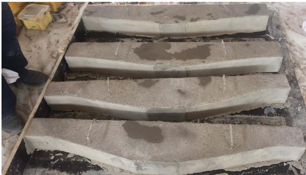
a. Removing formwork after casting
