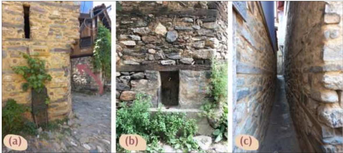
Figure 4.4: (a) Corner Chamfers / (b) Fountain / (c) Cin Street, Photographed by (Author, 2024).
