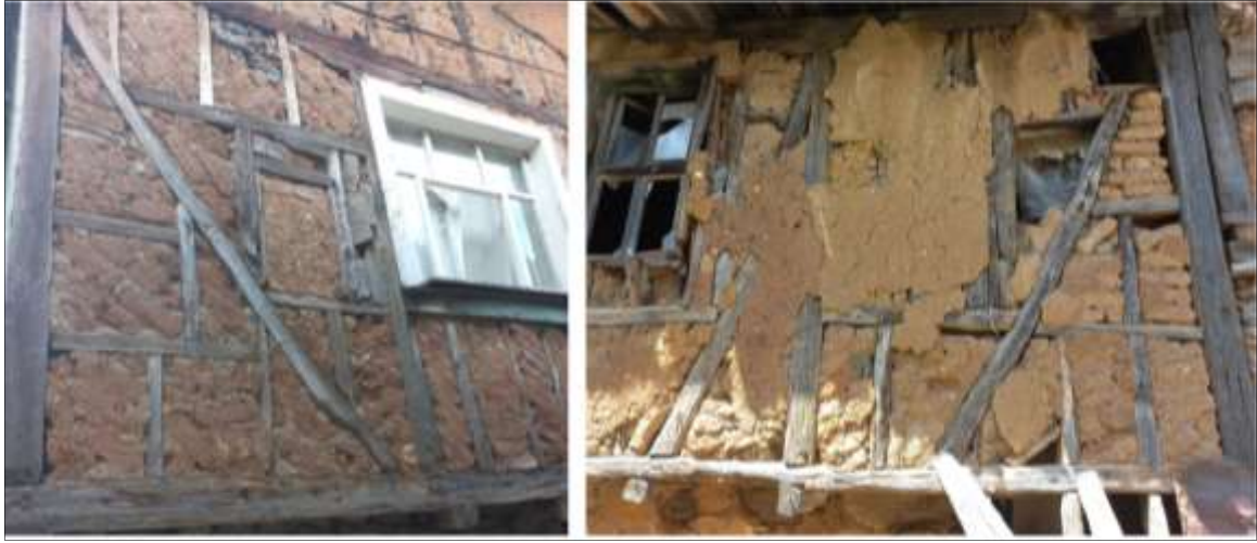
Figure 4.15: Adobe Fill Material Between the Wooden Framework in Cumalıkızık Houses.
