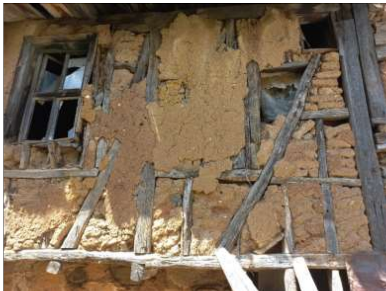
Figure 4.21: Example of the Usage of Plaster and Adobe in Cumalıkızık.
