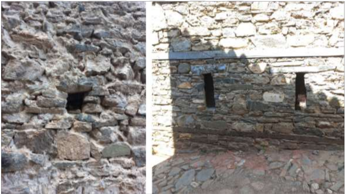
Figure 4.13: Ventilation Openings, Photographed by (Author, 2024).
