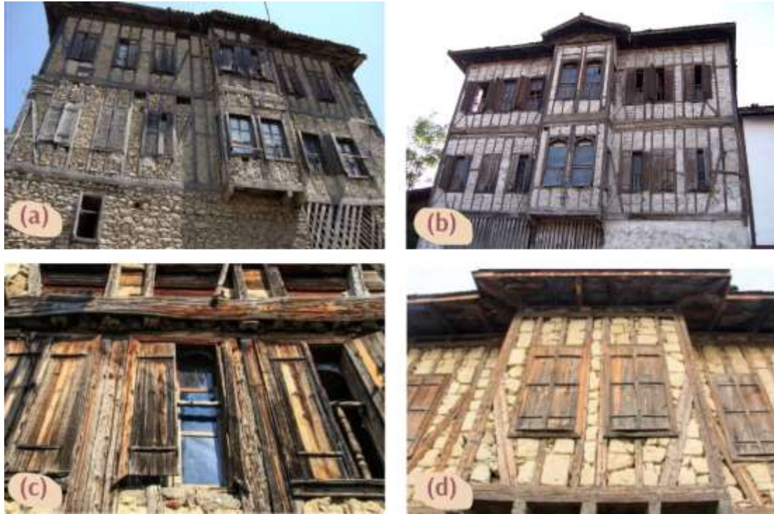
Figure 4.40: Examples of Facade Walls in Safranbolu (a) & (d) Stone Filled Walls, (b) Adobe Filled Walls, (c) Wood Filled Walls (Flickr Search — “safranbolu.” n.d.).
