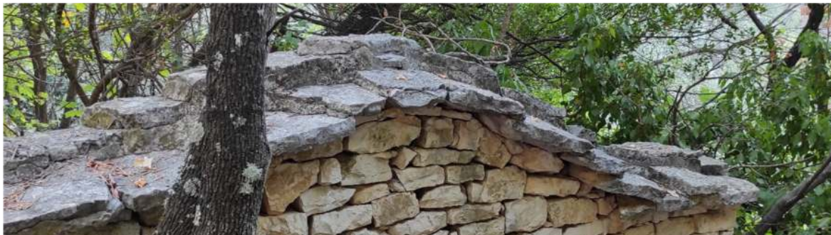
Figure 4.2: Dark gray stone slabs for roof cover.
