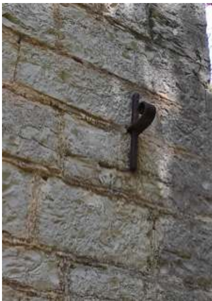
(Left) Figure 4.10: Cast iron masonry fastening. Detail from a 'tzineti.'
