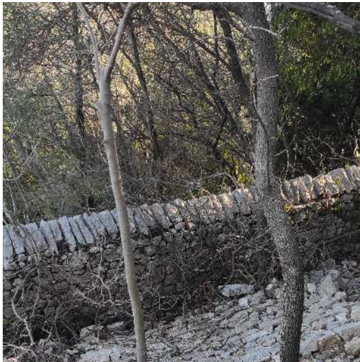
(Left) Figure 4.12: Ovoros with inclined stone slabs covering the wall premises/ samari . (Right) Figure 4.13: Courtyard gates.
