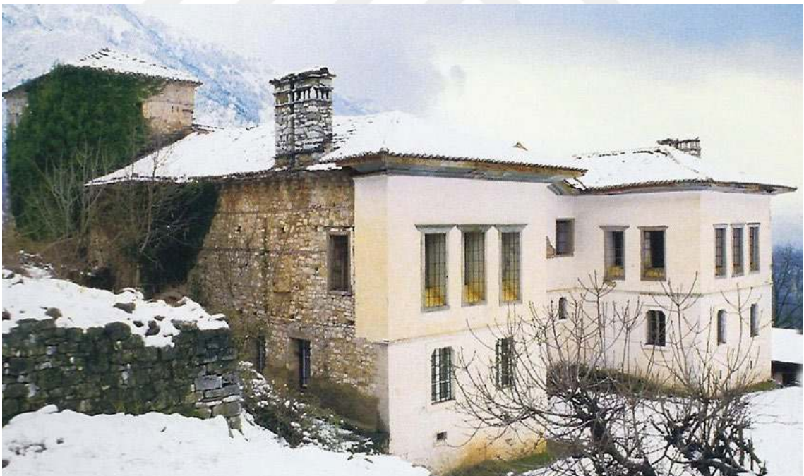
Figure 7.21: Sisko's house in Konitsa. Photo before its collapse. https://www.konitsa.gr/visit/othomanika-mnimeia-9/6-arcontiko-cousein-mpee
