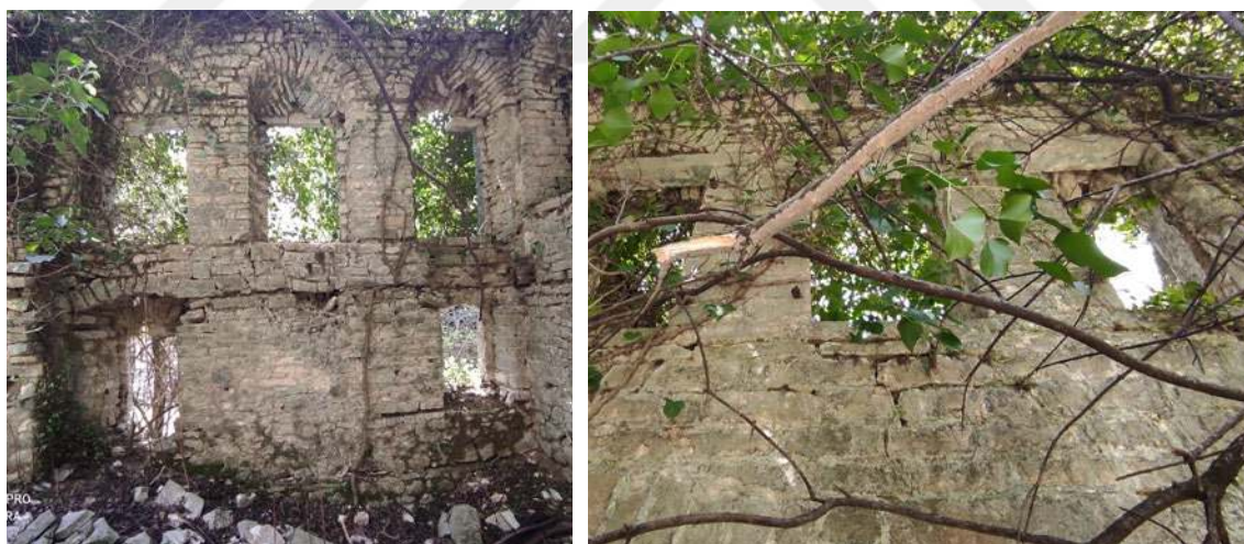
(Left) Figure 4.148: Interior south facade of the Household 14.
