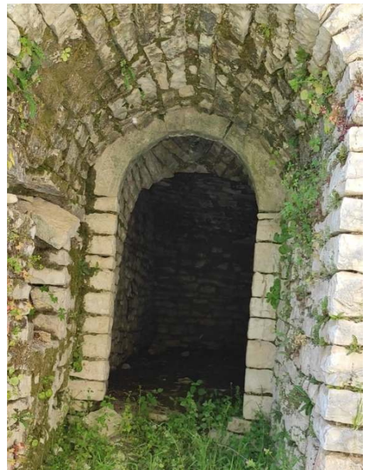
(Left) Figure 4.46: Door lintel with monolithic lintel and lowered pressure relief arch.
