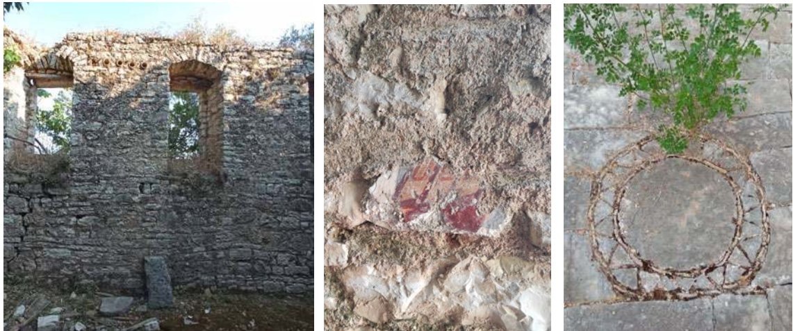
(Left) Figure 5.13: South wall from the interior of Aghios Dimitrios. Note the decorative ceramic mouthpieces.
