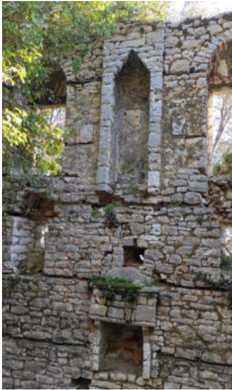
(Left) Figure 4.16: Fireplace substructure in the masonry/ kalokairino /southern room. (Right) Figure 4.17: Fireplace with rectangular escalating volumes in the masonry of a katoi / north room
