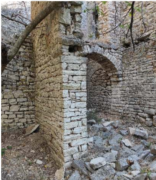
(Left) Figure 4.34: The L-shaped alteration with an enclosed entrance.
