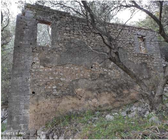
(Left) Figure 4.36: Typical façade, rendered with mortar- well-curved corner stones. (Right) Figure 4.37: Interior walls' render with a final, colored grinding layer.
