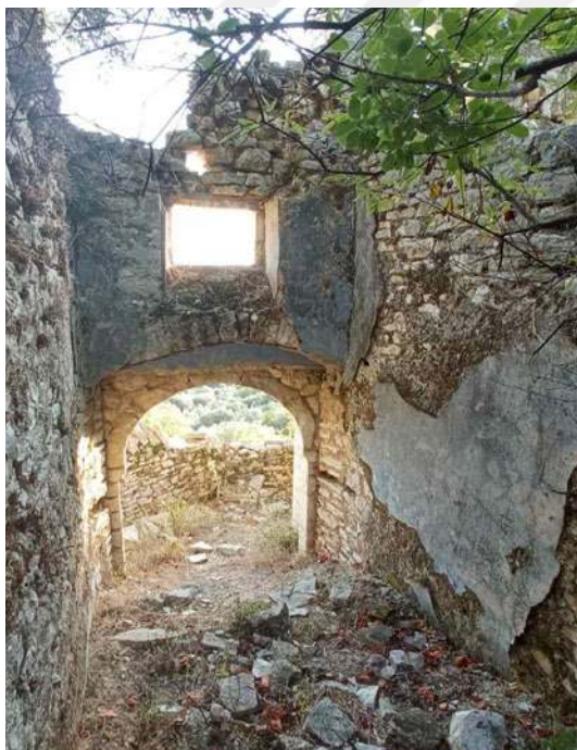
(Left) Figure 4.85: Interior facade of the lobby.
