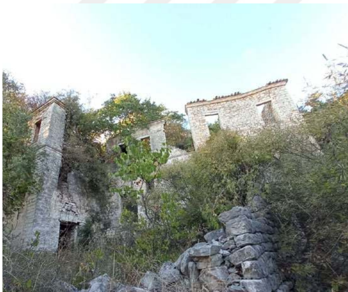
(Left) Figure 4.69: General south view.
