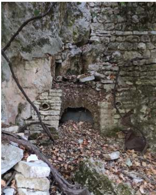
(Left) Figure 4.26: Furnace structure. Of notice are the ventilation ceramic mouthpieces.
