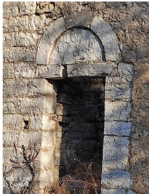
(Left) Figure 4.42: Window with monolithic lintel and lowered pressure relief arch.
