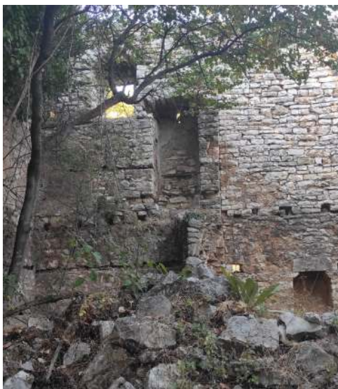
(Right) Figure 4.18: Niche at the vaulted area beneath the outdoor stairs - varelopithoma (Left) Figure 4.19: Cupboard substructure and niches on the east wall of a house.
