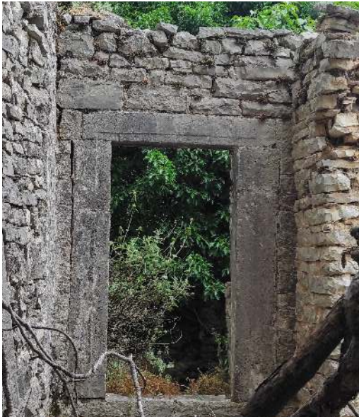
(Left) Figure 4.48: Door with monolithic lintel and stone jambs.
