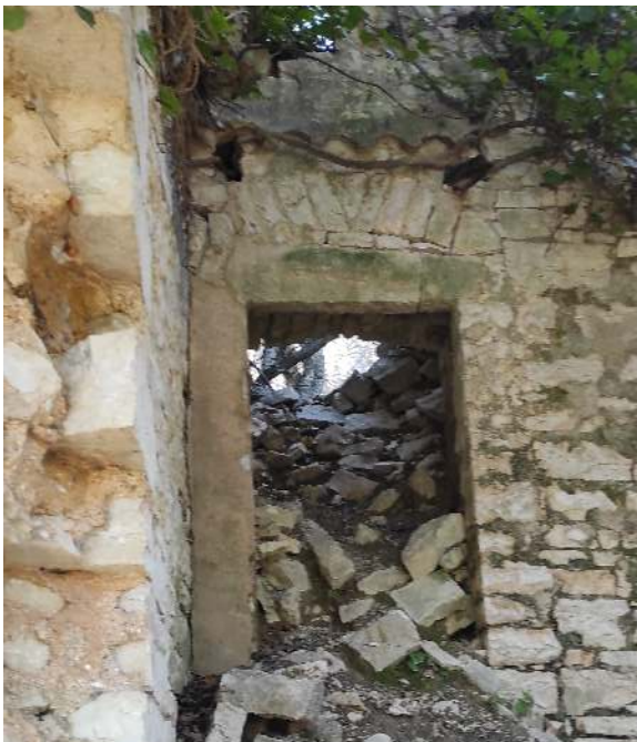
(Left) Figure 4.46: Door lintel with monolithic lintel and lowered pressure relief arch.
