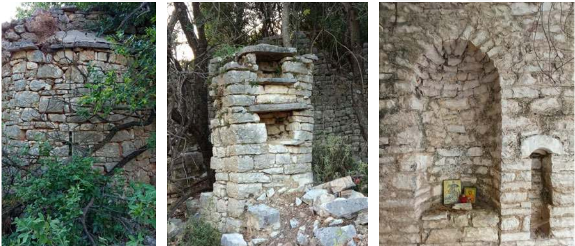
(Left) Figure 5.21: Exterior facade of Aghios Spyridon's apse.
