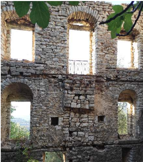
(Left) Figure 4.44: Window lintel structures with barrel vaults and lowered arches.
