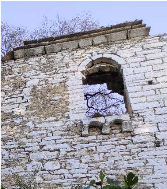
(Left) Figure 4.40: Protruding window aprons seating on stone corbels.
