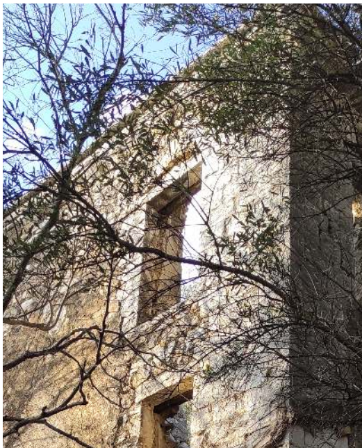
(Left) Figure 4.42: Window with monolithic lintel and lowered pressure relief arch.
