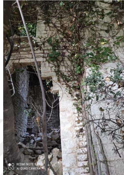
(Left) Figure 4.107: Littel protrusion leaning on a corbel-like base: From the the skylight of the house's main entrance.
