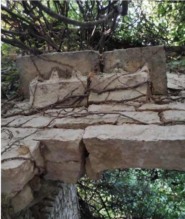
(Left) Figure 4.107: Littel protrusion leaning on a corbel-like base: From the the skylight of the house's main entrance.
