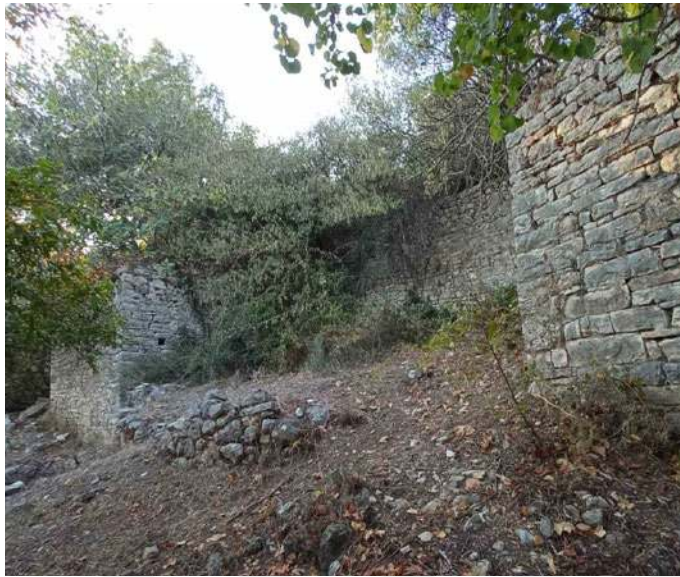
(Left) Figure 4.67: South courtyard wall.
