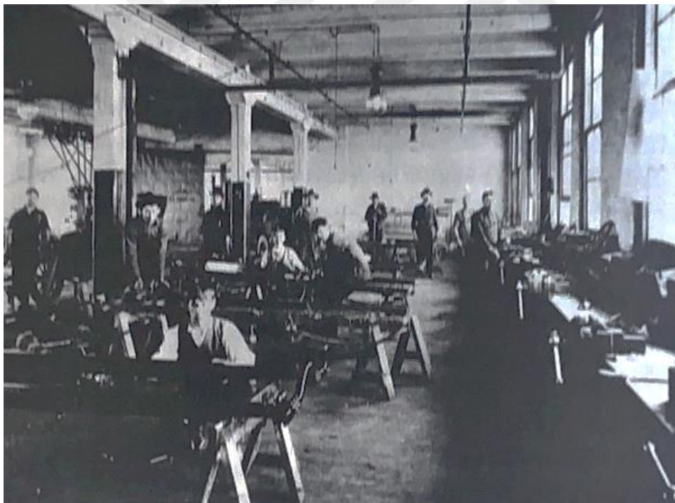
Figure20. Interior organisation of Piquette Avenue Factory, workers in an electrified room and producing by pre-assembly line technologies.
