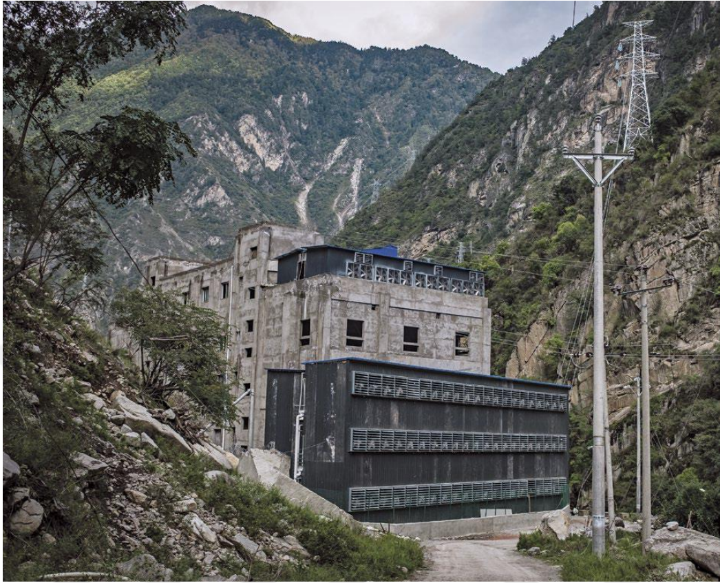
Figure43. Photograph of the outer view of the Bitcoin mine building, taken by Liu Xingzhe in 2016.
