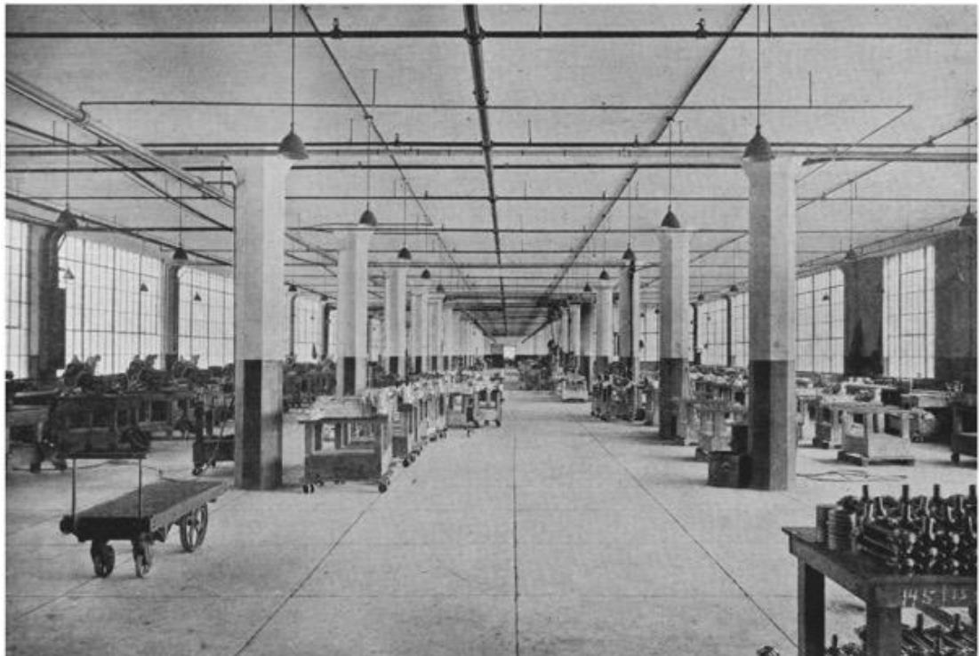
Figure22. Interior view of the assembly department of the Packard Motor Company Works, Albert Kahn, 1917. Layout of a daylight factory in the absence of workers, window-walls naturally illuminating the work environment, wide spans with reduced number of columns to open up more space, electrical lighting arranged as supplementary according to a grid, pipes were organised at the upper layer and invisible configuration of electrical wires that uncluttered and simplified the assembly hall. Structurally simplified, generic base of a nth plan of this daylight factory modelling the common variation of the typical plan.
