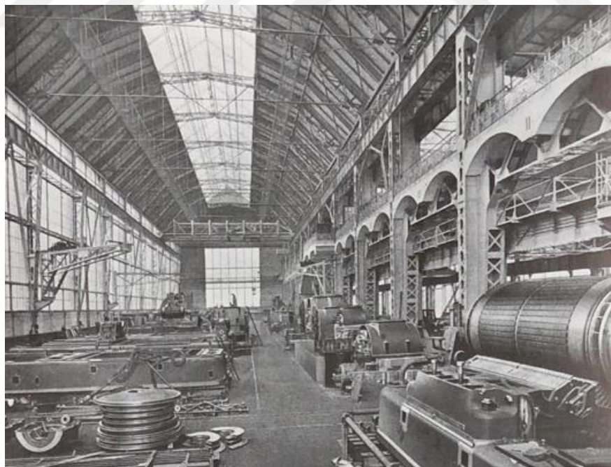
Figure15. Interior View of the Main Assembly Hall of the Turbine Factory. Modular replacement of machineries with prominently visible iron structure and utilisation of glass inside the factory.
