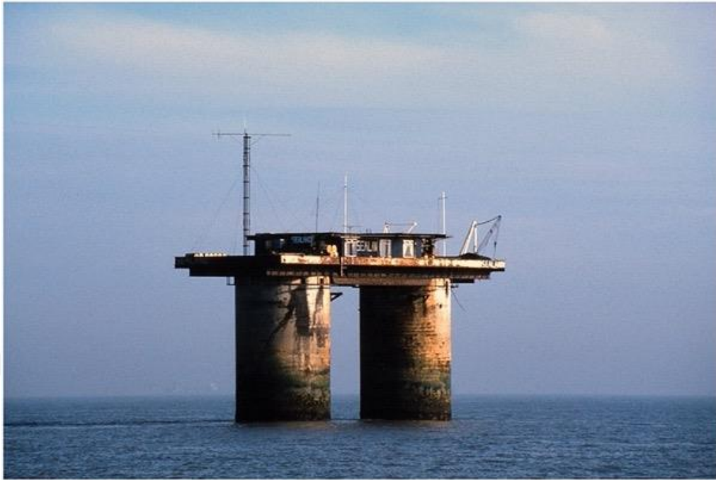
Figure39. Photograph of the Principality of Sealand, taken in 1986 by John Wray, showing two concrete legs supporting the main deck with a single storey building and helipad on the roof the building.
