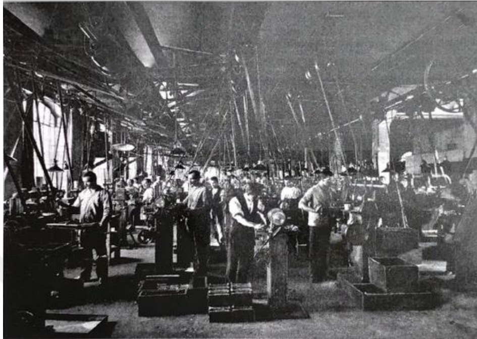
Figure11. Photograph of AEG Appliance Factory in Ackerstrasse (1888-95), showing a workshop powered by mechanical transmission. The confluence above workers with the transmission and lighting appliances is visible.
