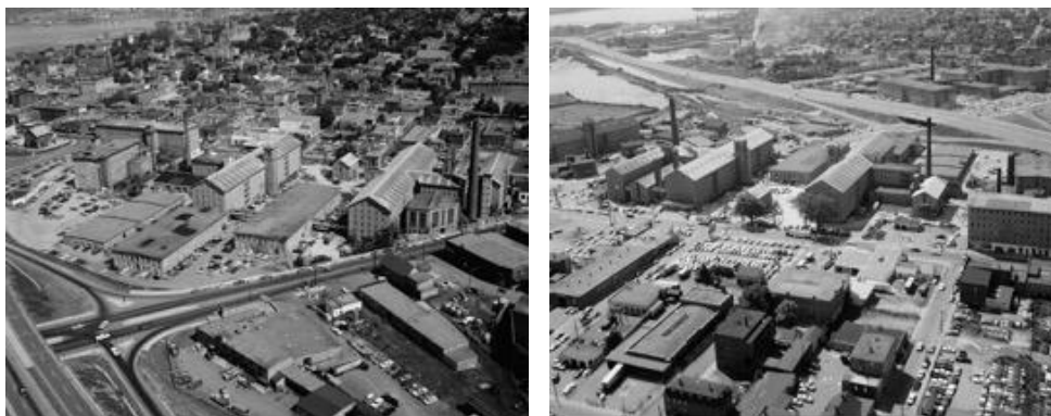
Figure8. Aerial Photographs of Durfee Mills, August 1968, Toward North (left) and Southeast (right) capturing all buildings with their surrounding environment.
