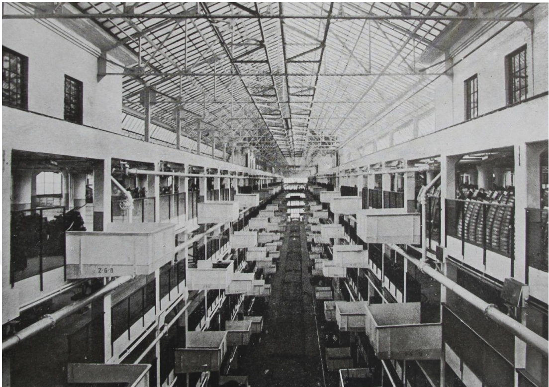
Figure26. Inner Configuration of the New Shop with electrical cranes, balconies in various levels, and railroad tracks at the bottom to carry products to the shipment area after production completed.
