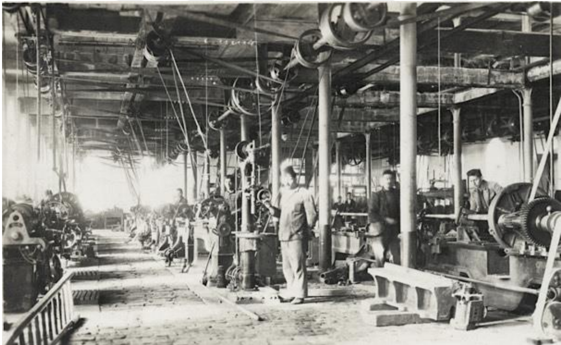
Figure37. Interior view of the production space under the Administration of Seyr-i Sefain in 1920s, before Istanbul Chamber of Commerce, and Ford Motor Company Exports Inc. Mechanical gears, shafts, and belts were supported through steel columns and opened the production space.
