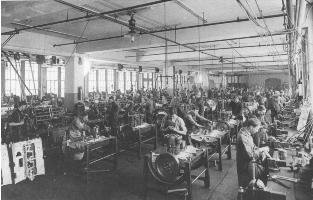
Figure21. Interior view of Packard Motor Company Building Number Ten, Albert Kahn, 1905. Earlier interpretation of a daylight factory, in spite of set electrical fixtures, some gears, belts, and shafts were still in-use, workers closely aligned at workstations in front of large windows.
