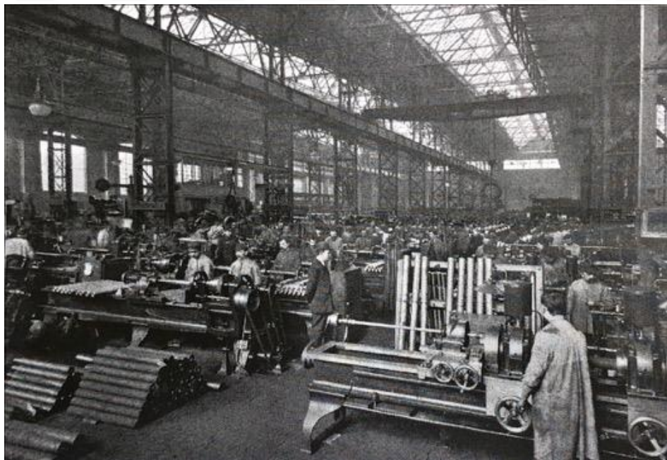
Figure12. Photograph of AEG Large Machines Factory in Brunnenstrasse (1895-97), showing a workshop powered by electrical single motor drive.
