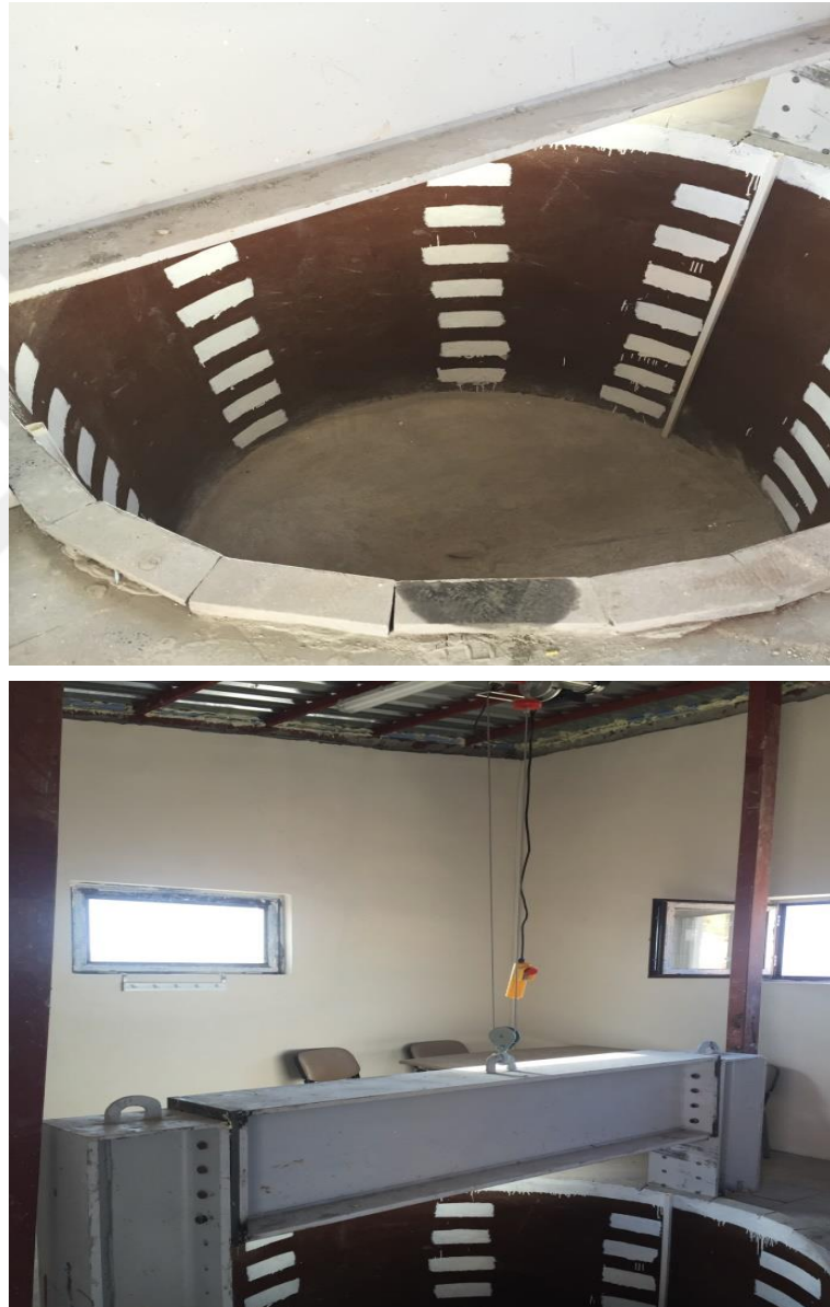
Figure 3.6 Box and frame used for plate load test
