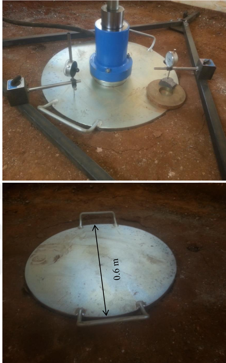
Figure 5.37 Failure shape for DAPs at the end of plate load test
