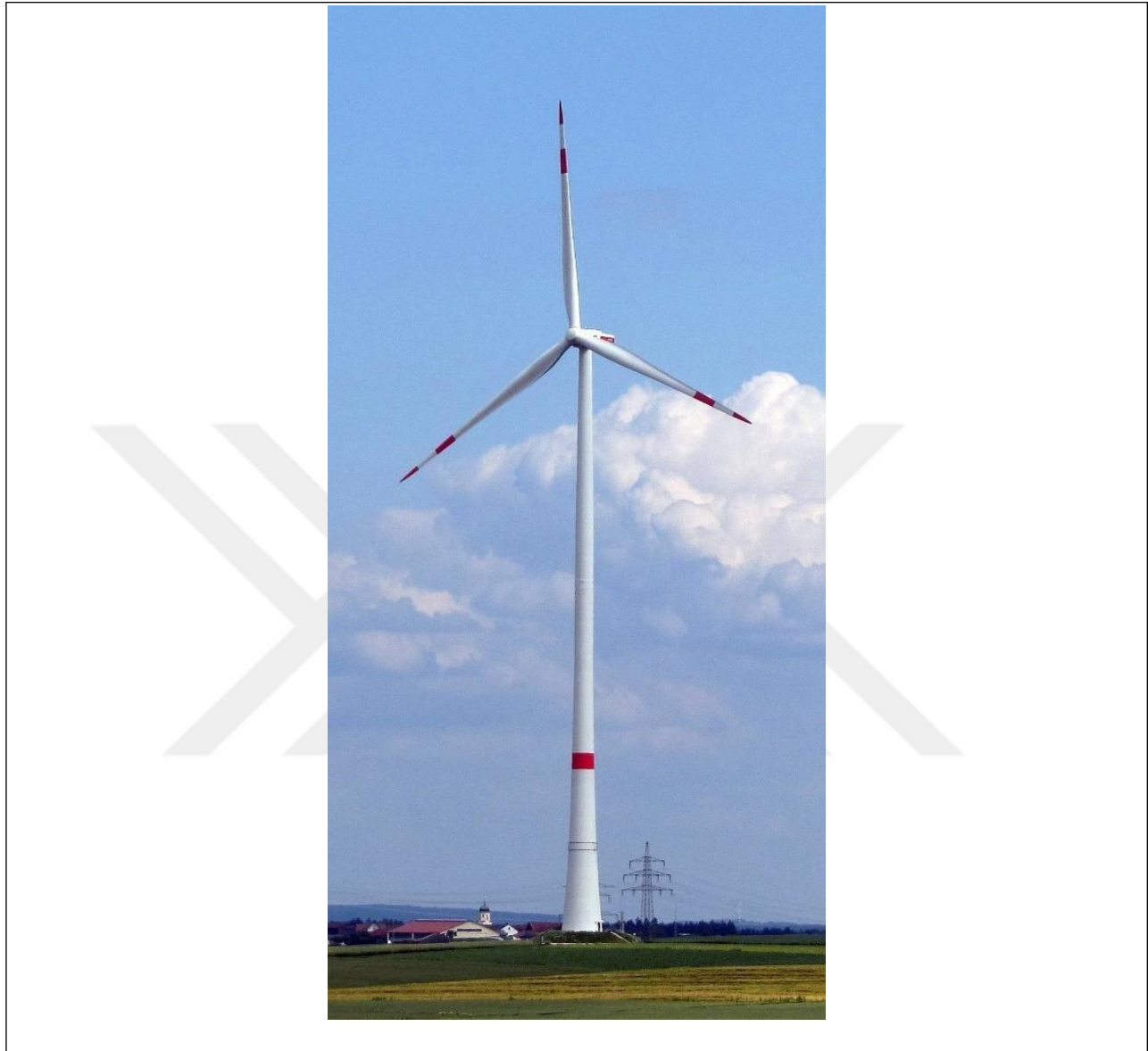
Figure 2. 3: Modern (2013) Wind turbine of the 3 MW class
