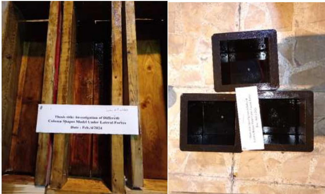
Figure 3.2: Oiling The Molds.
