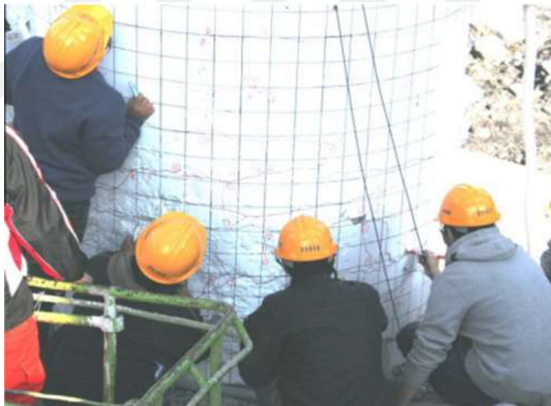
Figure 2.2: Cracks Manually Marked Using a Pen.
