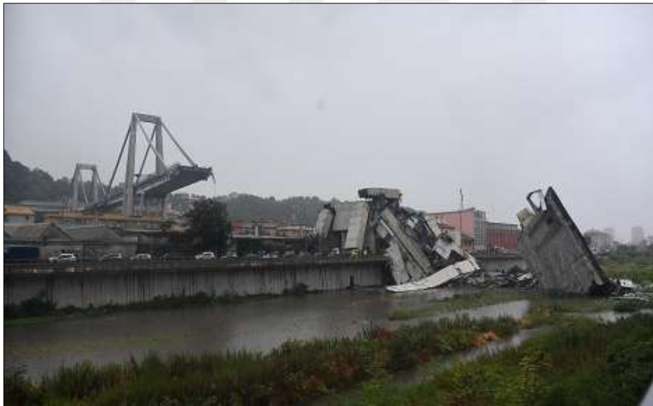
Figure 1.1: Morandi Bridge Collapse Incident.
