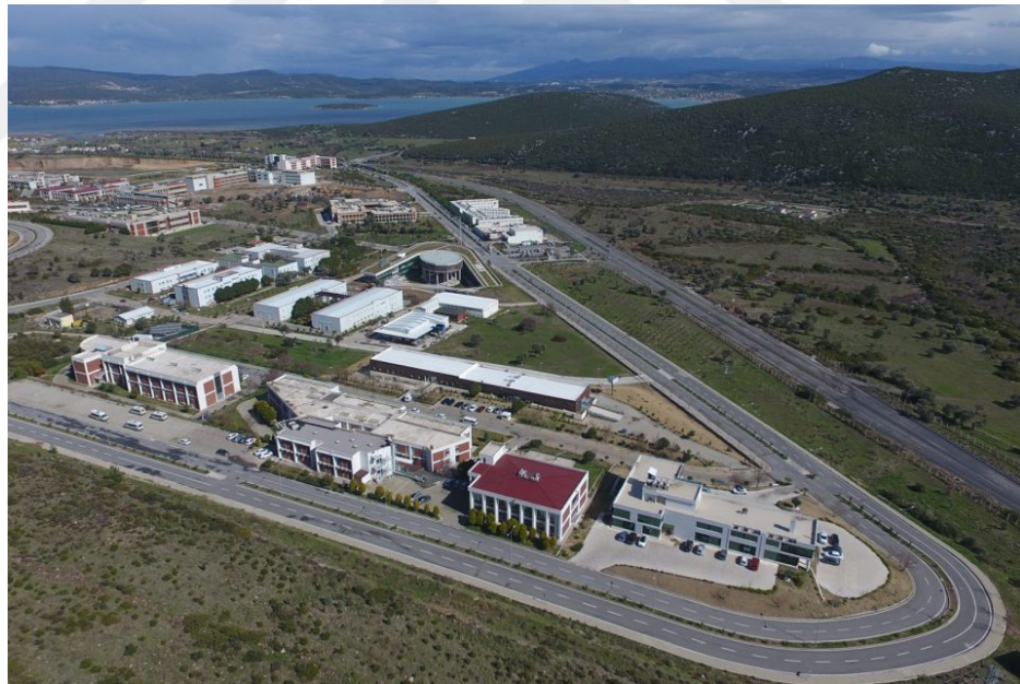
Figure 3.23 : Technopark region (Source: IYTE website)
