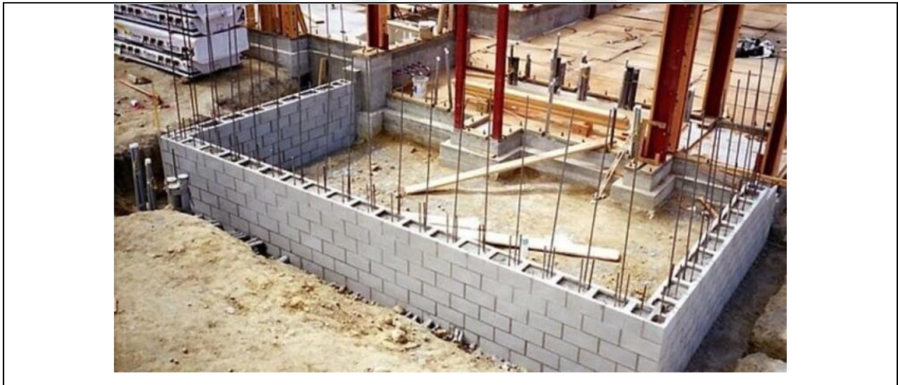
Figure 2.23: RC Hollow Concrete Wall Masonry
