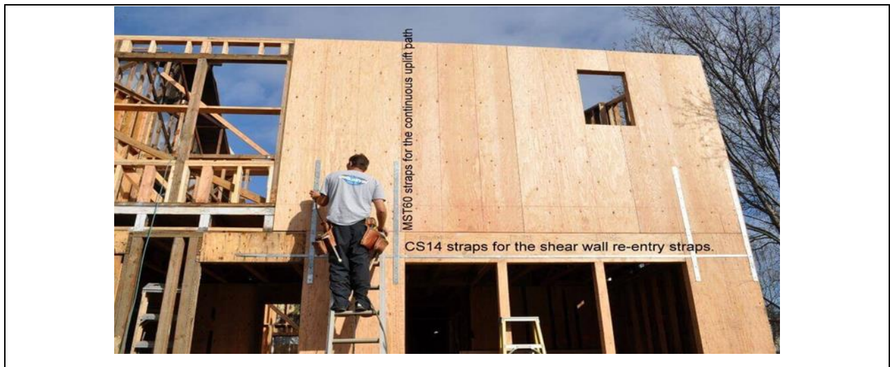
Figure 2.22: Plywood Shear Wall
