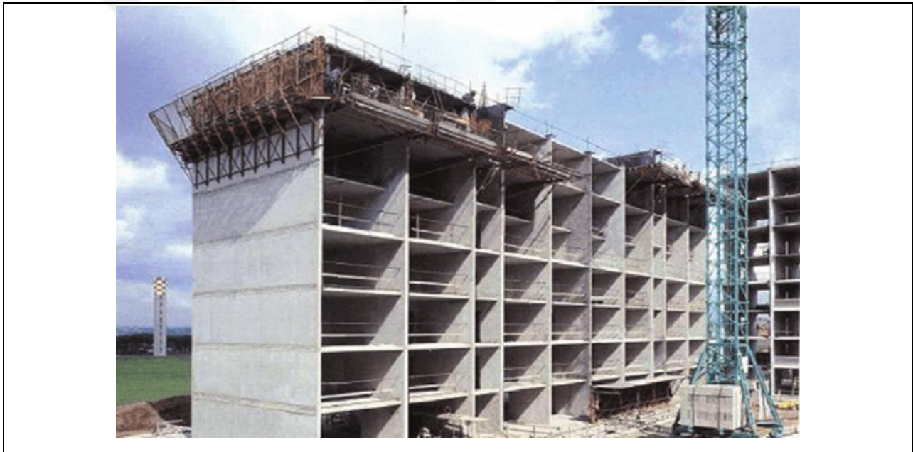
Figure 2.20: Concrete Block Shear Wall
