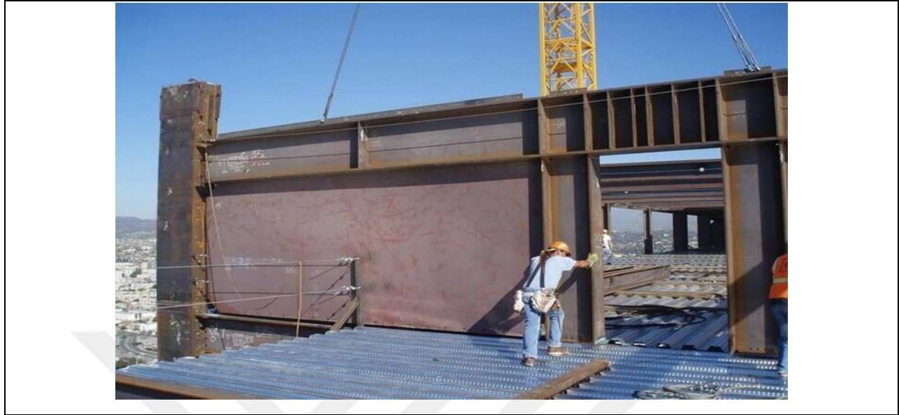
Figure 2.21: Steel Shear Wall
