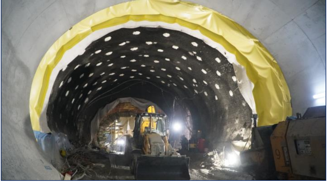
Şekil 3. 3. NATM (New Austrian Tunneling Method) ( https://www.tunelmarket.com/blog/natm-tunel-metodu )
