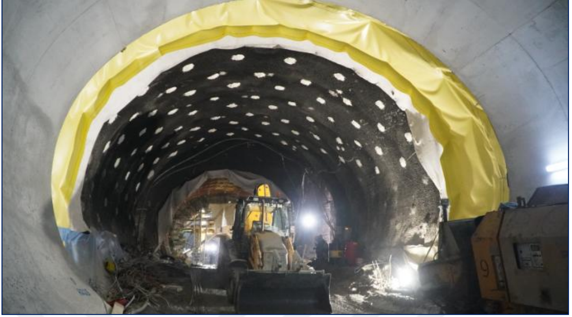
Şekil 3. 3. NATM (New Austrian Tunneling Method) ( https://www.tunelmarket.com/blog/natm-tunel-metodu )
