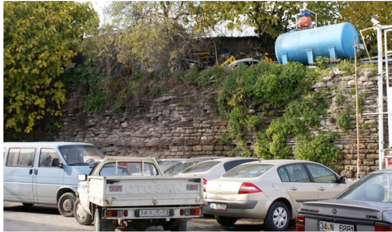
Fig. III.30. View of the harbor's remaining walls lying on the western part of the tower, Ercan 2009.
