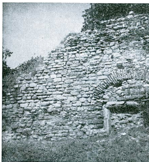
Fig. III.28. View of the gate next to the tower 65.
