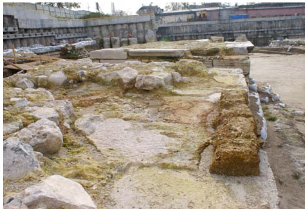
Fig. III.49. Detail of the bricks on top of the dock looking to south, Ercan 2008.
