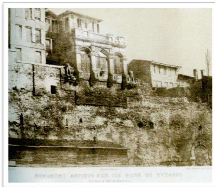
Fig.I.14. The seawalls along the Marmara shore, photo. by Trémaux.
