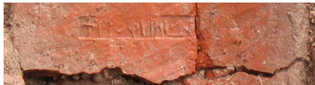
Fig. III.35. Structure No.5, detail from the brickstamps, Köşker 2005.
