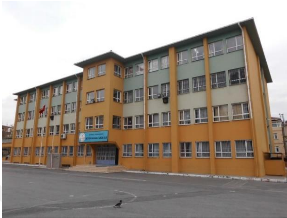
Figure 4.1. Outside view of the investigated Büyük Halkalı Primary School building
