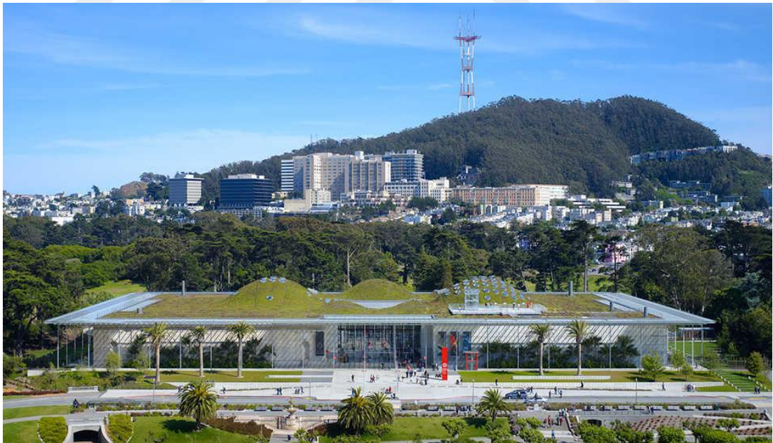
Figure 8. General view of California Academy of Sciences. ( https://www.calacademy.org/efficient-daily-operations )
