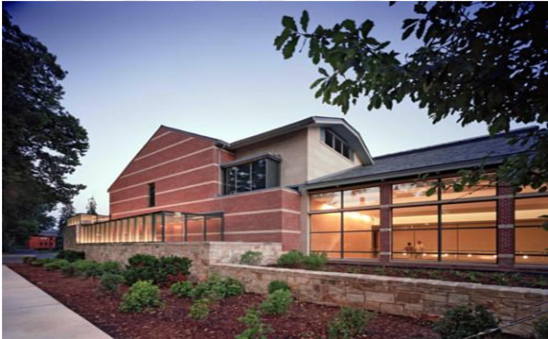
Figure 6. Mark Twain Historic House and Museum, One of the earliest LEED certified museums in the world.
