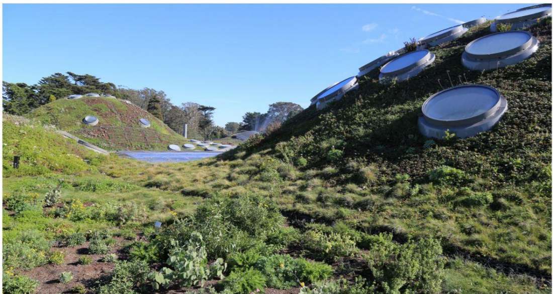
Figure 10. The green roof of CAS with native Californian plants. ( https://www.calacademy.org/exhibits/living-roof )
