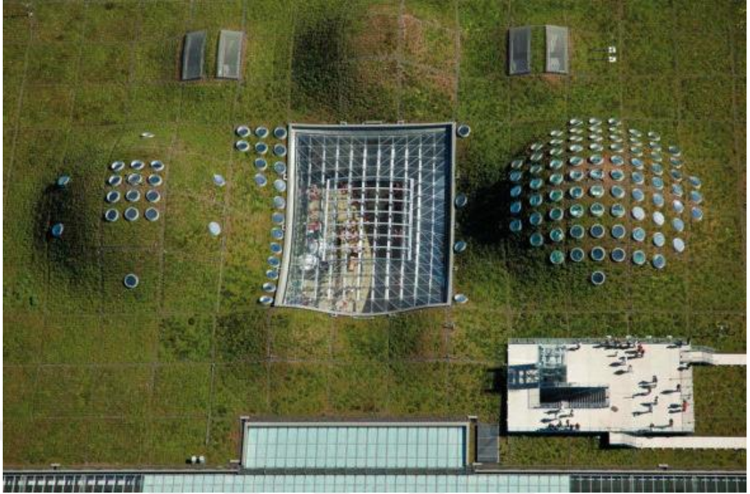
Figure 11. The air view of the CAS's roof. ( https://arch-com.net/en/architectural-articles/908cec16-california-academy-of-sciences#images-gallery-11 )
