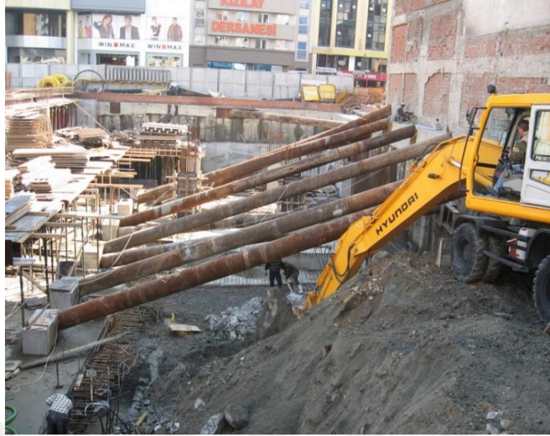
Figure 8.3 Steel pipe struts were added to give sufficient capacity to the shoring system and to limit the displacements
