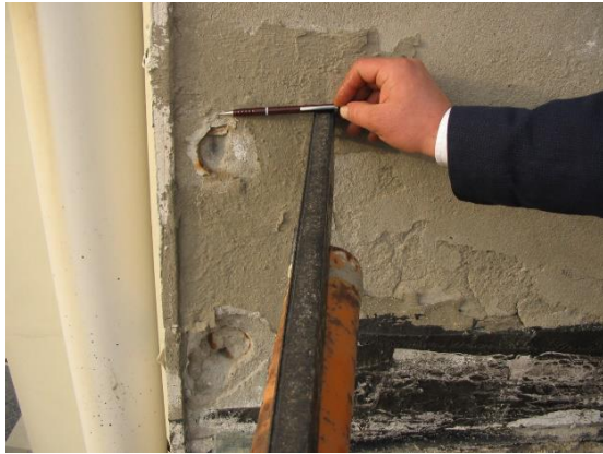
Deformation Perpendicular to the Excavation (14 cm)
