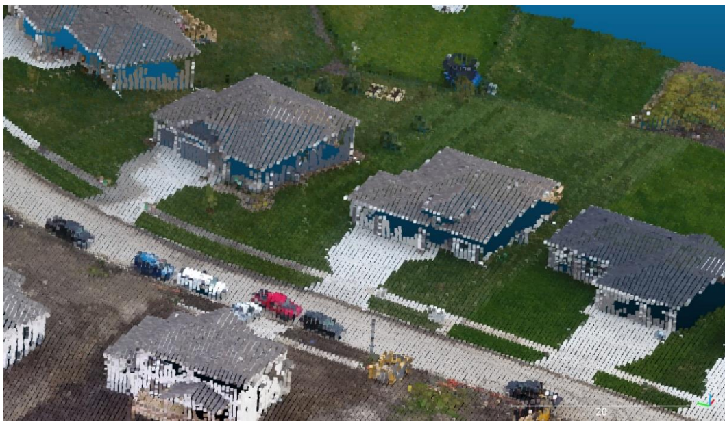
Figure 96: Missing points on facades
