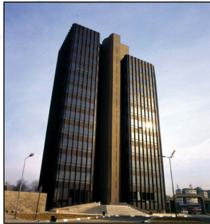
Figure 4.10. İstanbul Highways Zincirlikuyu Facilities [188].
