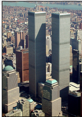
Figure 2.37. World Trade Center Buildings [107].
