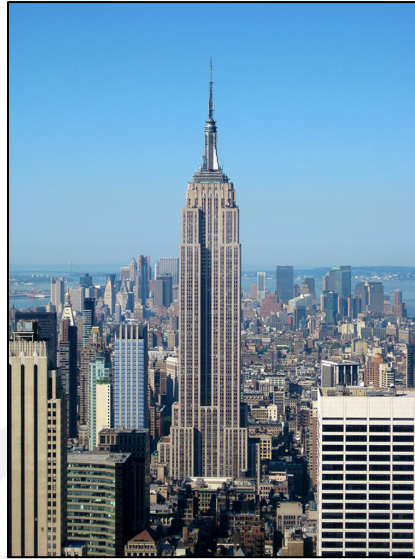
Figure 2.33. Empire State Building [99].
