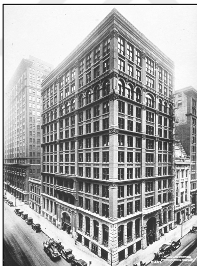
Figure 2.18. Home Insurance Building [78].
