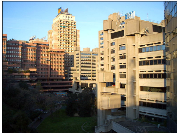
Figure 2.26. Torre Piacentini Building [90].
