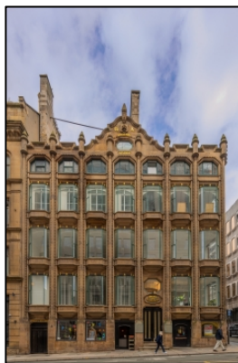
Figure 2.17. Oriel Chambers Building at Liverpool [73].
