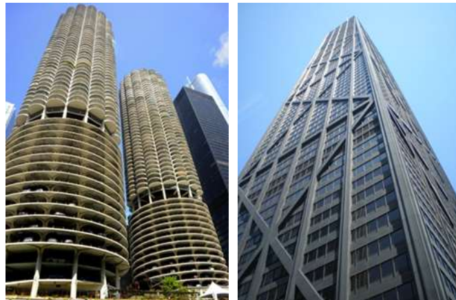
Şekil 2.11 (a) Marina City, (b) John Hancock Center (Archdaily, 2019)
