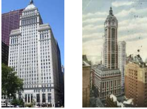
Şekil 2.8 (a) Metropolitan Tower , (b) Singer Tower (Mimdap, 2007)
