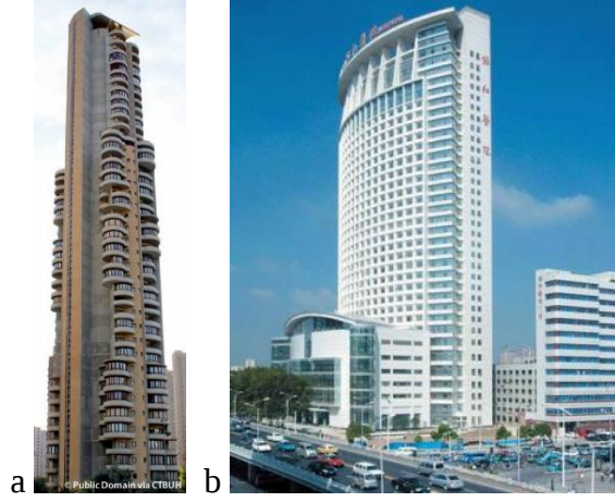
Şekil 2.5 (a) Edificio Neguri Gane (Skyscrapercenter, 2020) (b) Wuhan Xiehe Hospital Tower (Skyscrapercenter, 2020)
