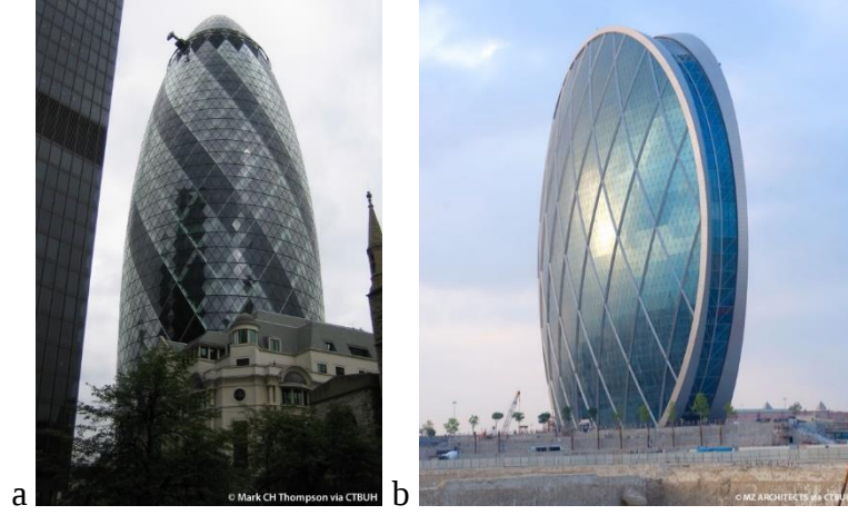
Şekil 2.7 (a) Swiss Re (skyscrapercenter, 2021) (b) Aldar HQ Binası (skyscrapercenter, 2021)
