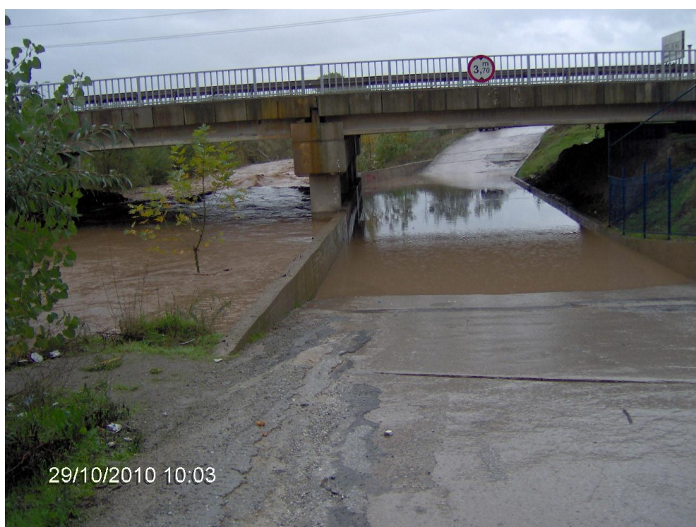
Figure 3.17 Downstream channel section at 11+400 km
